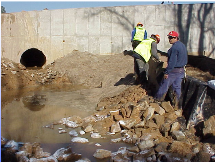
Above: The plunge pool collects the heaviest sediment discharged from underground storm drains.
