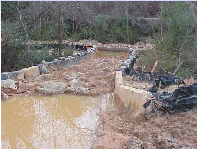
Above: The channel is a conveyance system that aids in the reaction of the Floc Log and APS Silt Stop treated storm water.
