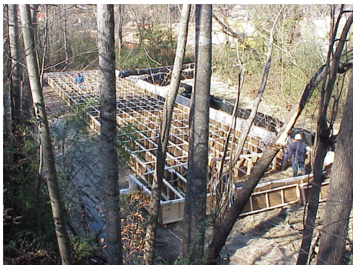
Above: The baffle grid is a system where phosphorus, inanimate particulates, pollution and sediments are flocculated out improving water quality and clarity.
